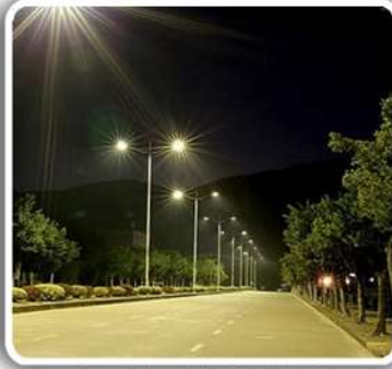
STREET LIGHTS & 24 HOURS ELECTRICITY
